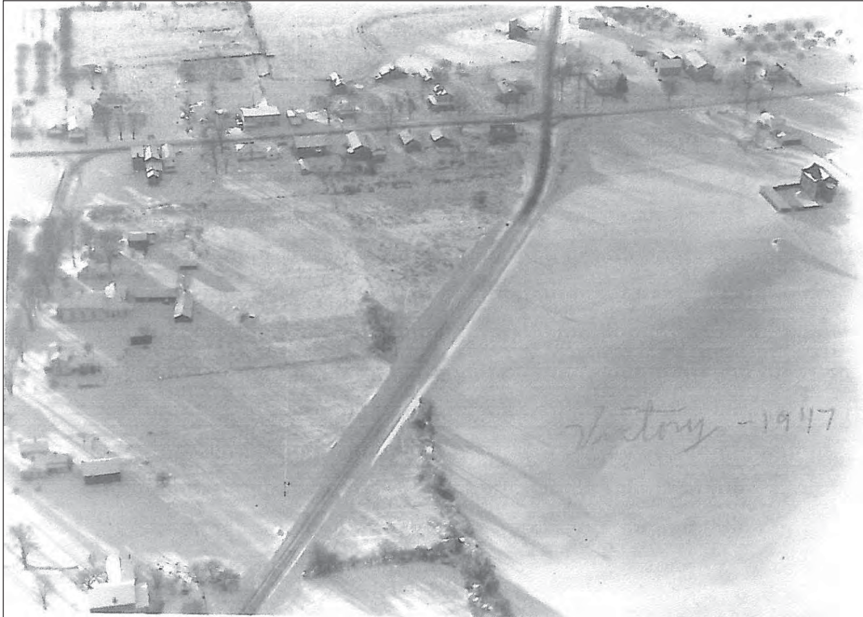
Aerial view looking west over the Hamlet of Victory in 1947, prior to the introduction of State Route 370.
